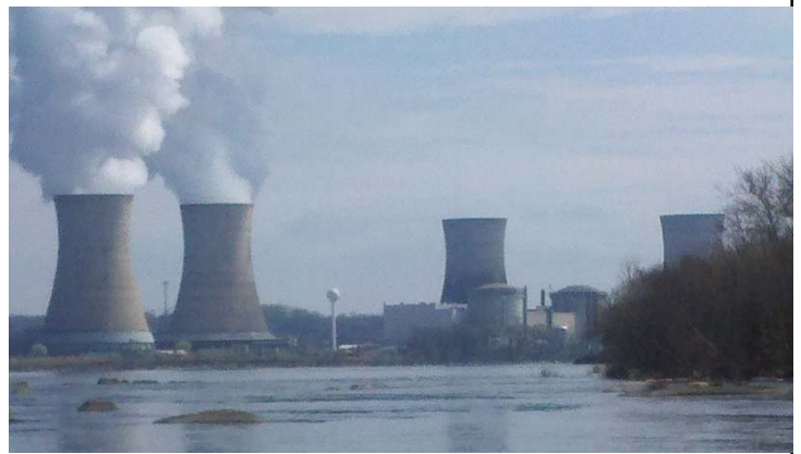
The Cooling Towers of Three Mile Island
